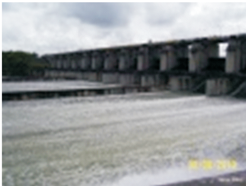
Fig. No. 1. Photo view of Pus Dam.
