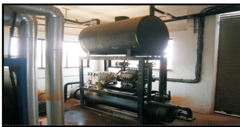
Photo Plate : 5. Filter and Drain
