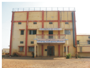
Plate-1 Puikhadee WTP located at 14km from the city on Kolhapur- Radhanagari road
