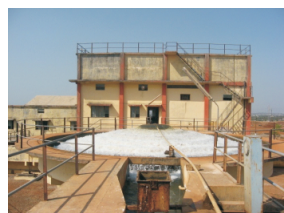
Plate-2 Aeration lagoon at Puikhadee WTP
