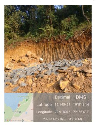
The bedrock is further cut and boulders are removed. These are used to construct gabion structures and at some places as landfill material. Excess material is removed at many places and the gaps between cut slope and gabion wall is filled with mucking generated. For this roads are constructed over the cuts as seen in following photograph.
