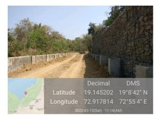
As there is cut and fill activity it is bound to create a steep slope which will be vulnerable to failure. The vulnerability is high especially due to high rainfall regime. To protect these newly created steep slopes gabion walls are constructed. The height of wall is indicator of the extent of cutting done at site. Following photograph shows the retention structure in form of gabion wall and the original slope marked on it.
