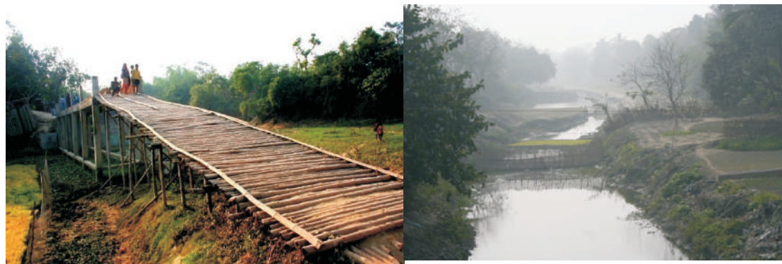
Plate 3. Obstruction along the river channel
